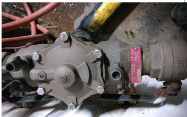
Figure 5: Backflow Preventer (Top View)
