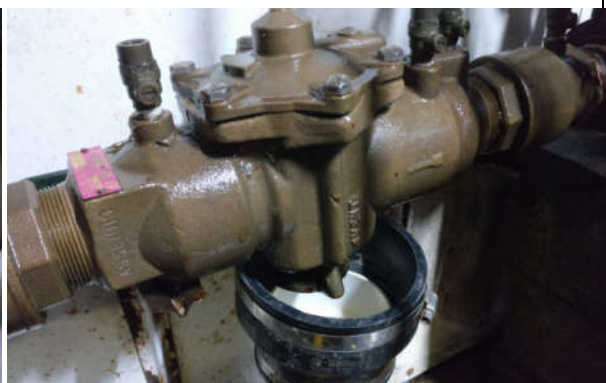
Figure 6: Backflow Preventer (Side View)
